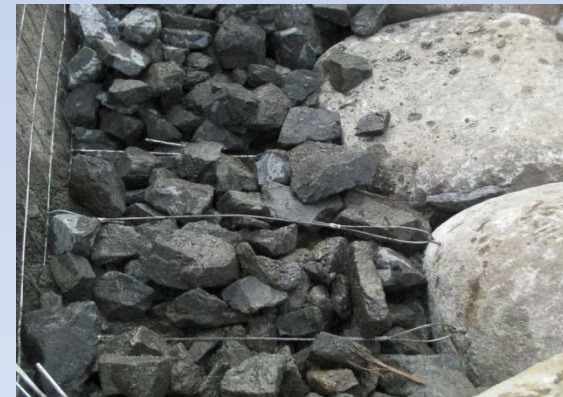
⑥裏込栗石敷き詰め
