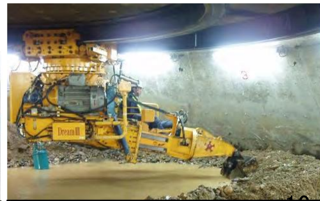
④掘削・沈設
